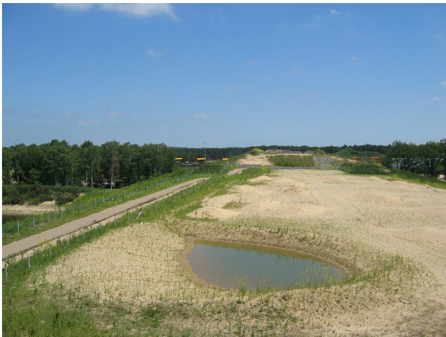
The overpass aims at facilitating migration of different species and therefore also includes watery elements (Source: Google Earth)
